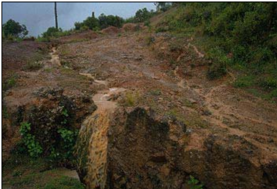
Photo 13.1 Do not leave disturbed or barren areas exposed to raindrops and runoff. Use erosion control measures to protect the area and protect water quality.
